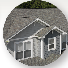
Roofing and Ventilation
